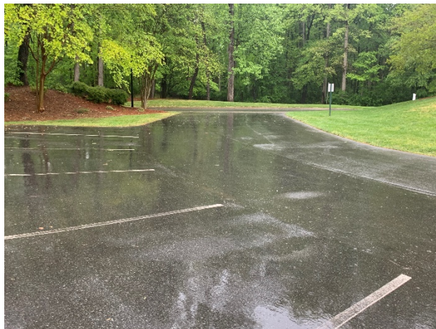
Parking lot overview
