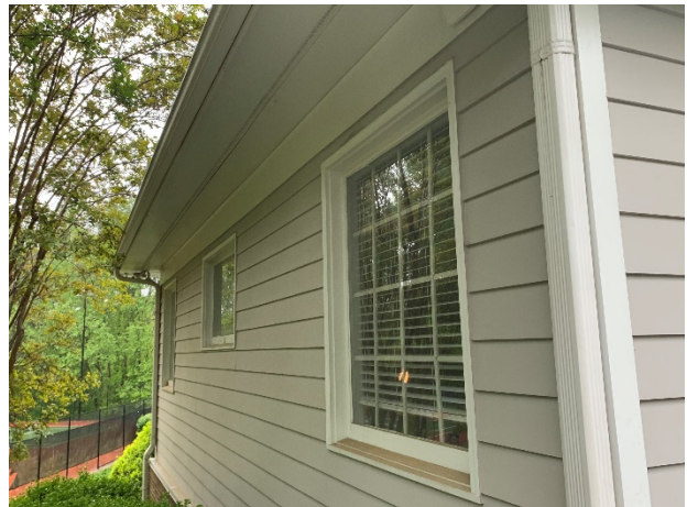
Paint finishes and sealants at the clubhouse
