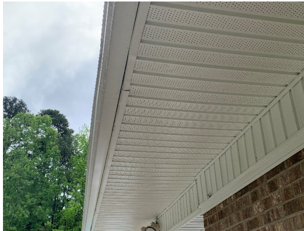
Vinyl soffit at the pool house
