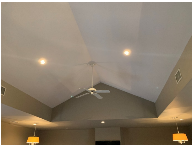
Paint finishes at the ceiling
