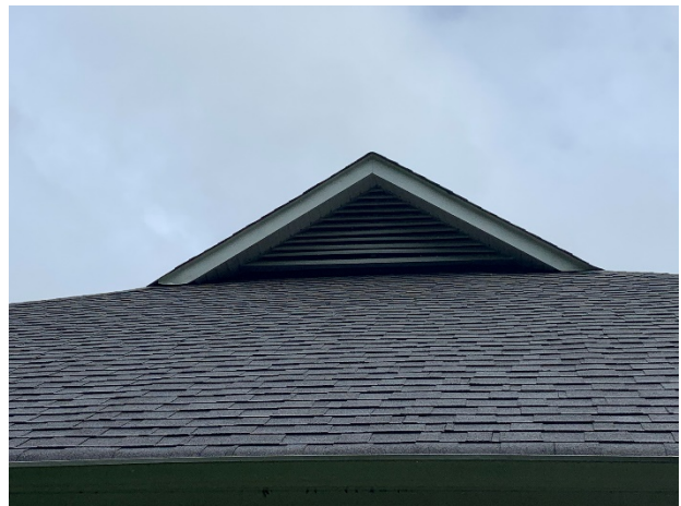
Asphalt shingle roof at the pool house
