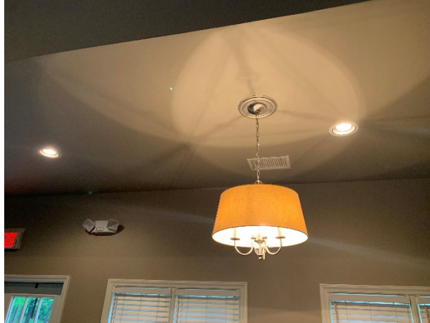
Ceiling and can light fixtures
