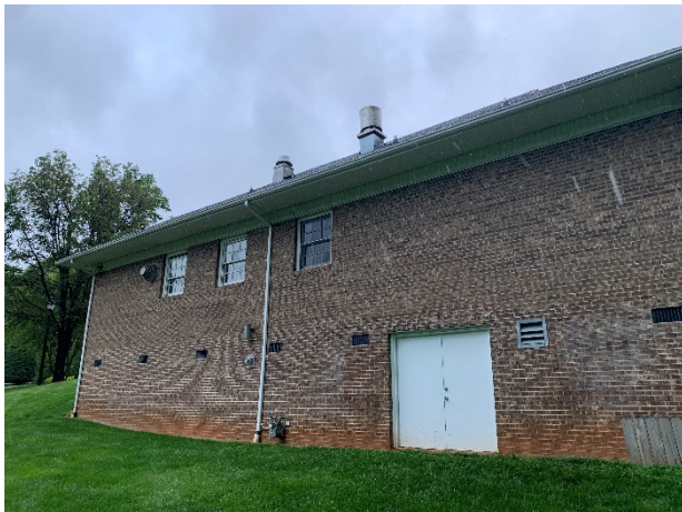
Rear elevation of the pool house
