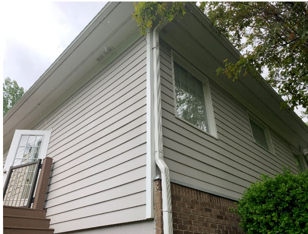
Downspout at the clubhouse
