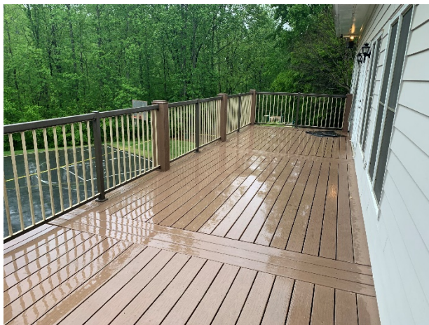
Deck boards and railings
