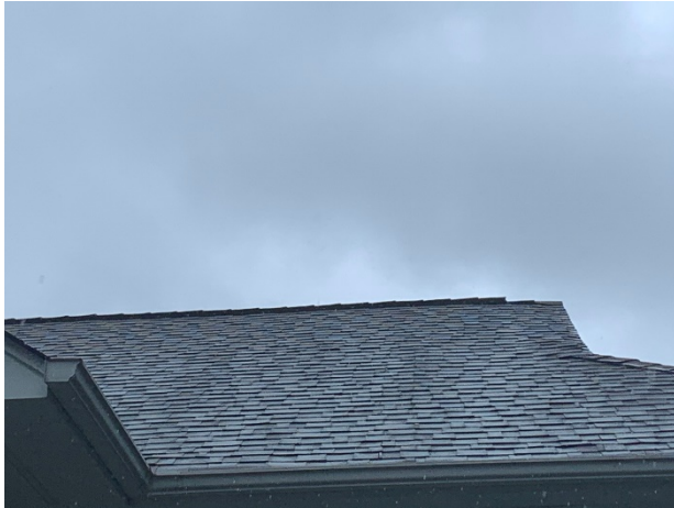
Asphalt shingle roof at the clubhouse
