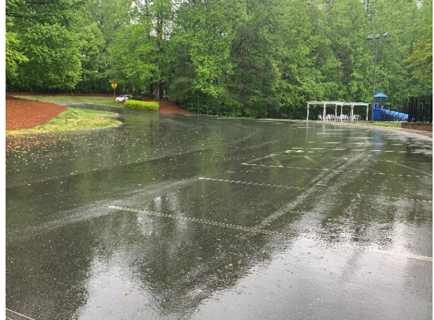
Parking lot overview
