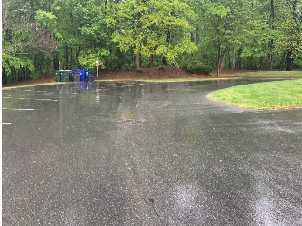
Parking lot overview
