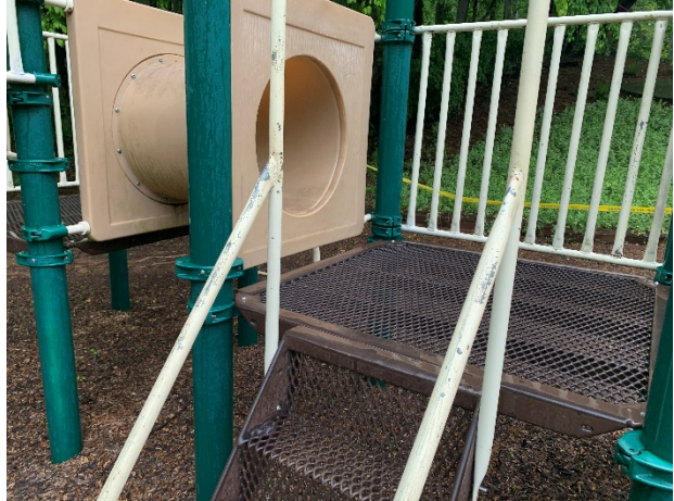
Finish deterioration evident
