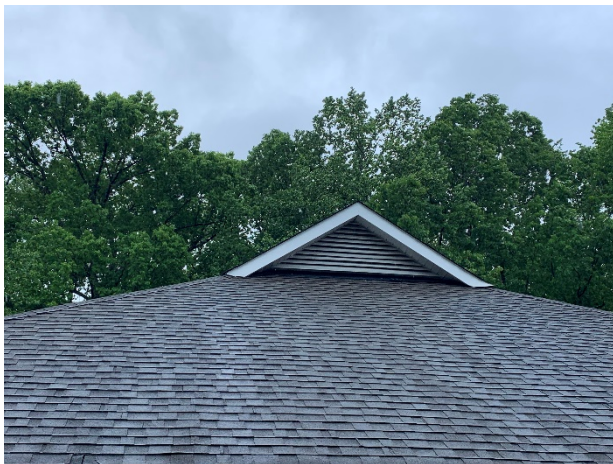
Asphalt shingle roof at the pool house
