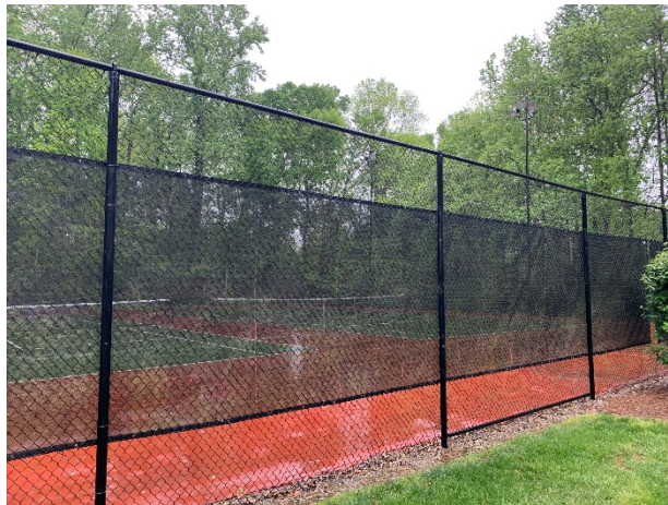
Tennis court fence
