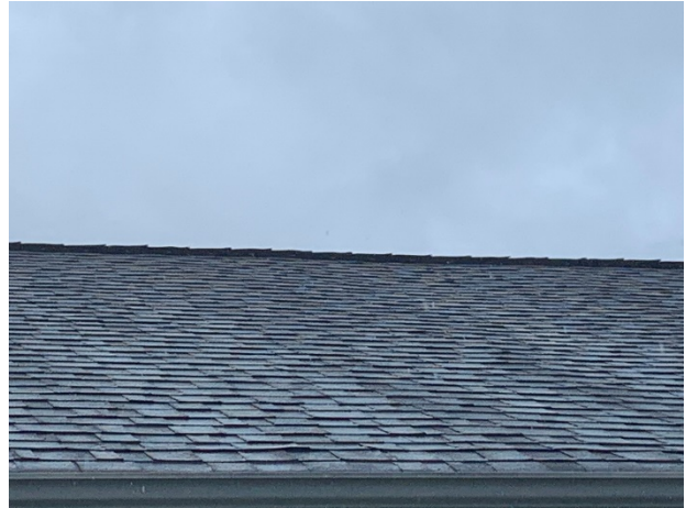
Asphalt shingle roof at the clubhouse
