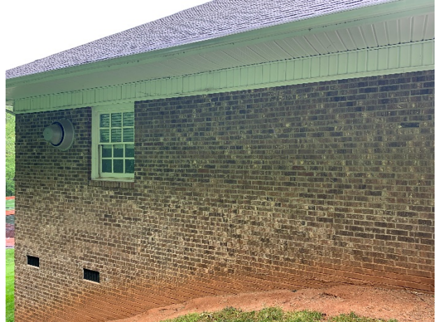
Masonry wall at the pool house
