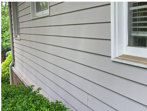
Side elevation of the clubhouse
