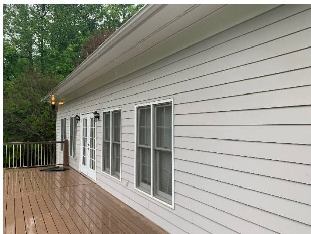
Rear elevation of the clubhouse
