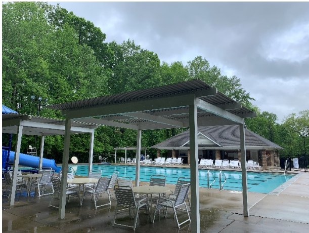
Shade structure overview
