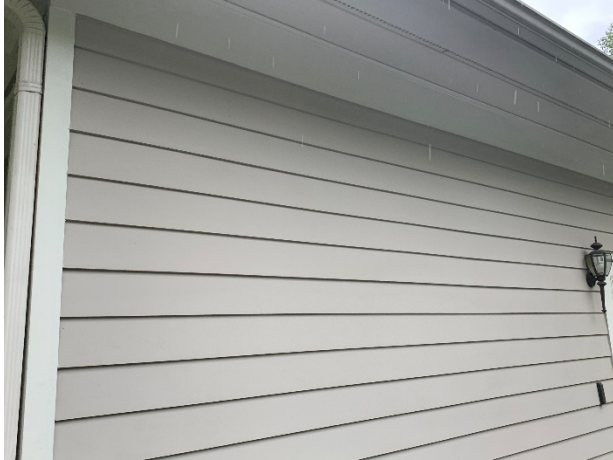
Composite hardboard siding at the clubhouse
